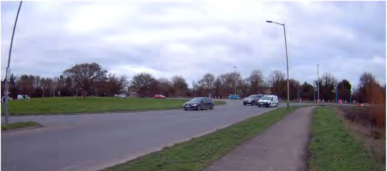
(View 3 – looking over the Bowerhill roundabout towards Melksham Town – A365 runs from right to left.)
